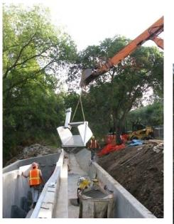
FlumeGate<sup>™</sup> slides into frame – next step is commissioning and then it is ready to pass water
