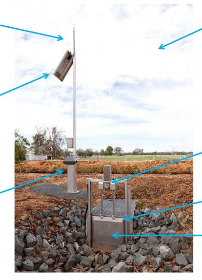
Highly accurate gate control  $\pm$  1/16 of an inch (positive actuation in both directions) Can run in following modes:
