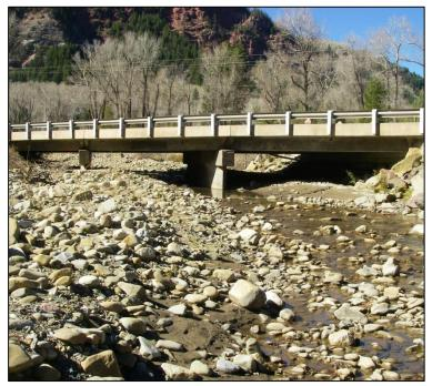
Figure 21. Coal Creek looking upstream. On the upstream side of the bridge the channel is highly modified, significantly down cut and no longer interacting with the floodplain or lower terrace. (RFC, October 2012)
