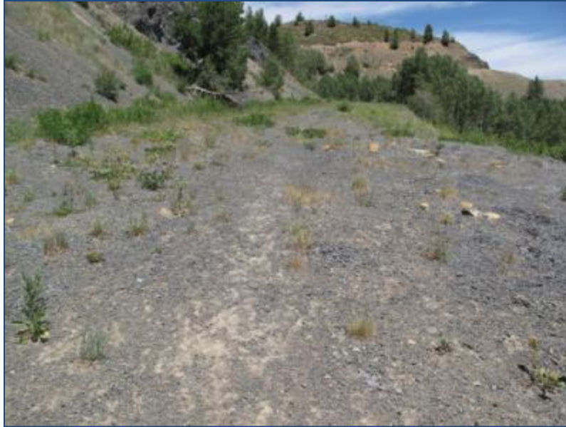
Figure 8. Road prism before treatment; road had minimal infiltration and excessive overland flow.
