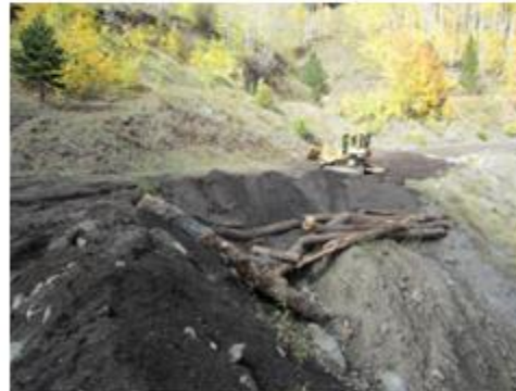
Figure 7. Area 2a during restoration.
