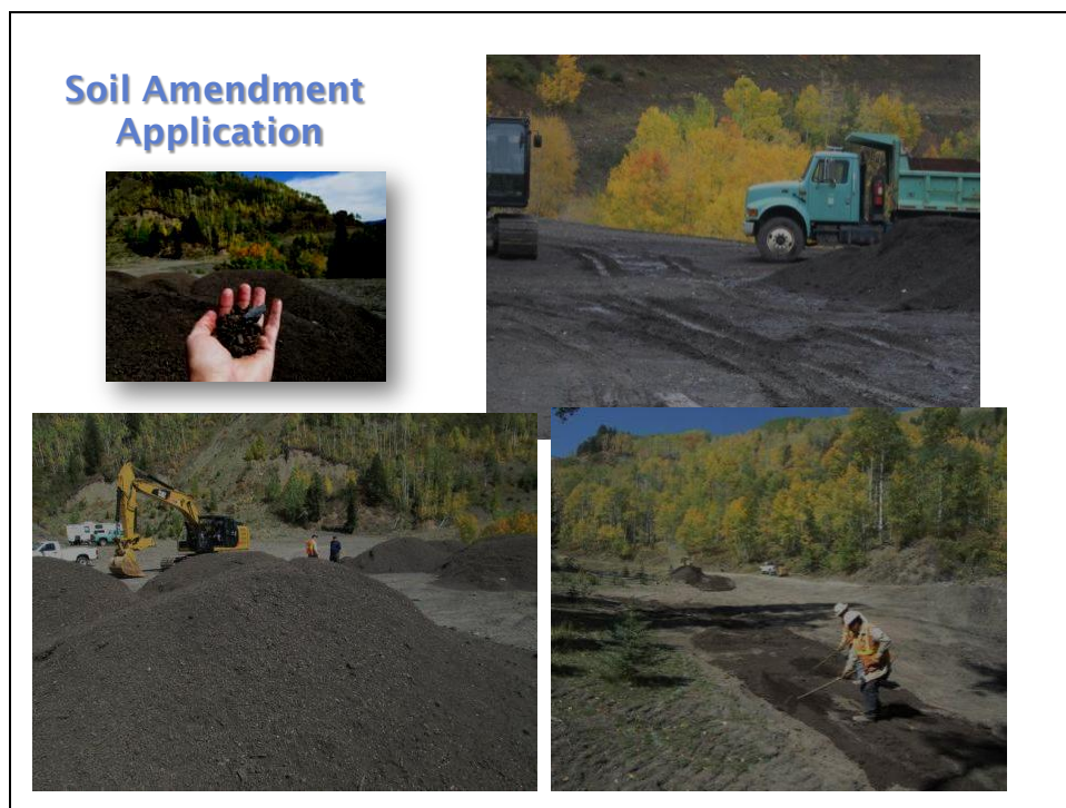
Figure 14. Application of biochar/compost and compost only soil amendments in treatment areas. Top left photo is a close up of biochar. Piles in photos are compost/biochar blend.
