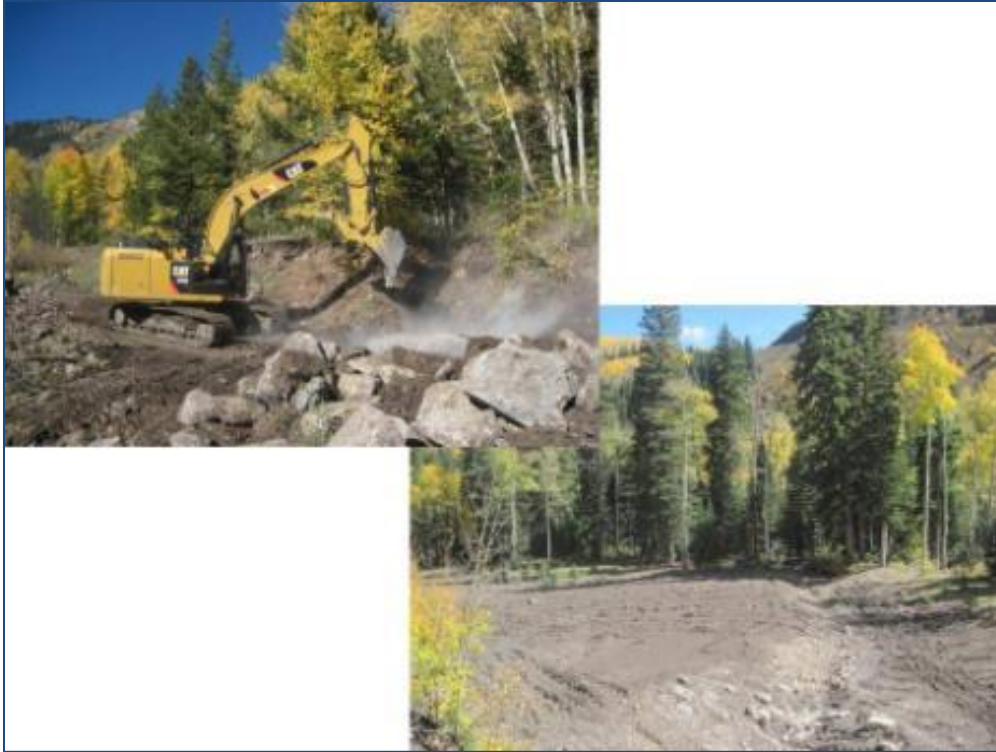
Figure 11. Area 2c alluvial fan during restoration.
