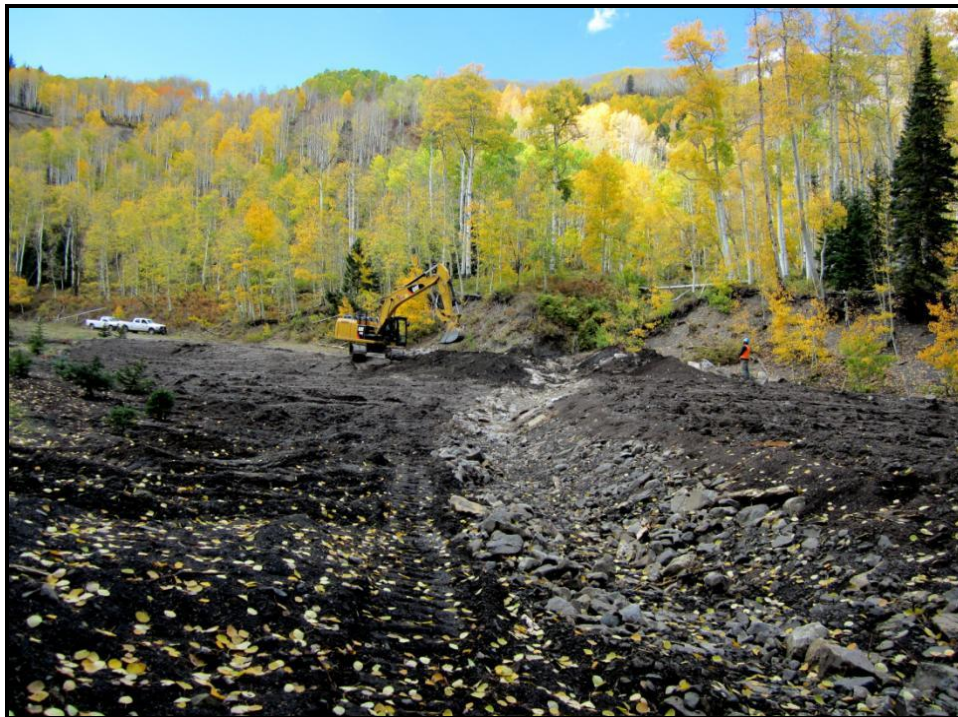
Figure 12. Area 2c alluvial fan during restoration.
