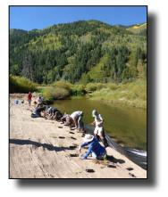
erosion control fabric, plant hundreds of native willows, install bank stabilization wattles, and re-seed the disturbed areas. The next time the river rises, these newly designed banks will allow the river to over-bank, thus slowing the flow, dissipating energy, and recharging groundwater. The new plants and erosion control measures will
