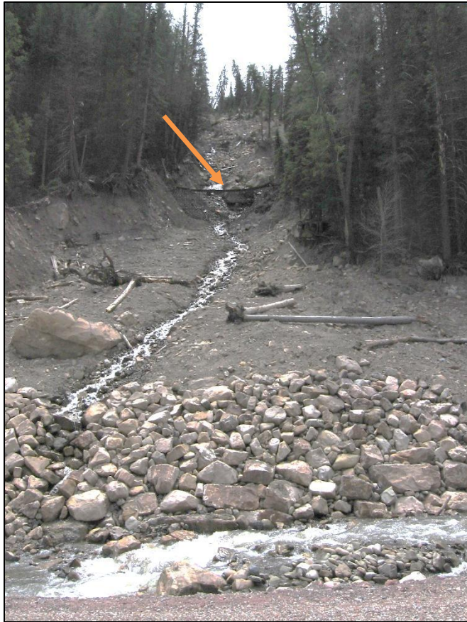
Figure 12. Debris flow near Braderich Creek trailhead with netting (at arrow) (May 1, 2012). The “toe” of the alluvial fan has been removed at the base.
