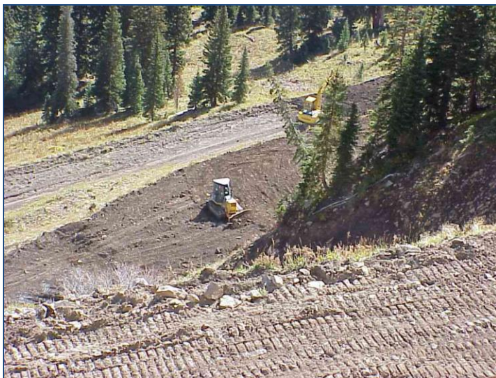
Figure 6. Road reclamation work in Coal Basin.
