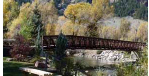
Pedestrian Bridge connecting Redstone and Elk Park
