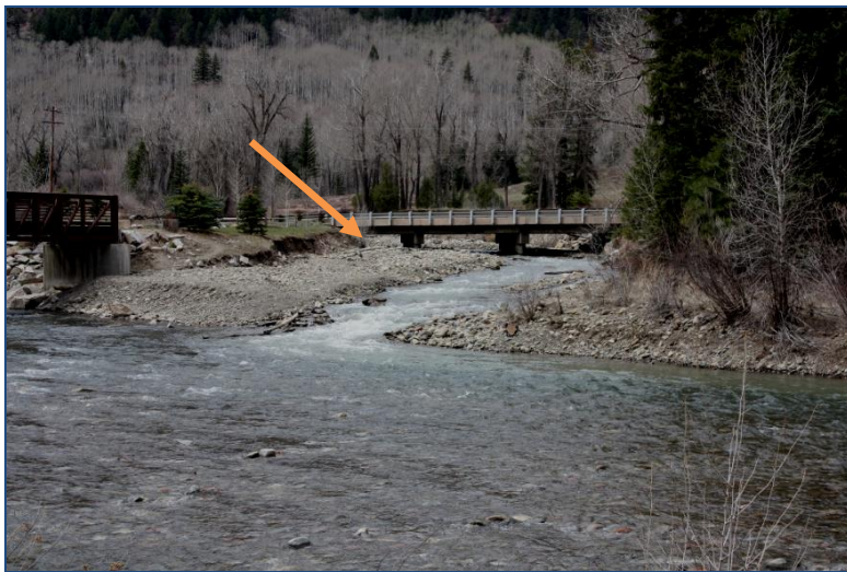
Figure 2. Coal Creek/Crystal River Confluence Area. Note the elevated gravel bars partially blocking clearance under the bridge.
