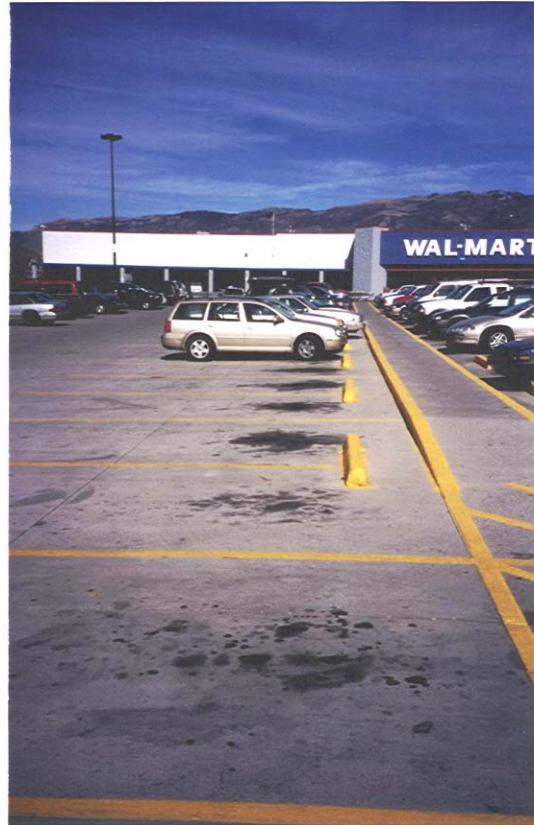
Figure 4: Presently, oils and greases from this parking lot are carried by stormwater directly into the storm drain system, and then enter directly into the Roaring Fork River, untreated. Phase II stormwater regulations require communities to explore ways to treat stormwater runoff.
