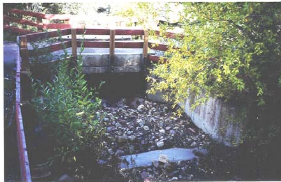
Figure 7: This drainage gully located on Red Mountain has been preserved to convey mud and runoff to the river. Maintenance is needed on a regular basis to remove accumulated rock and dirt and provide adequate conveyance capacity.
