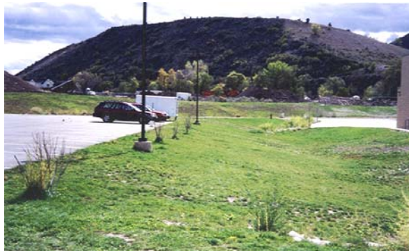
Figure 32: This surface detention site around the new Sopris Elementary School is a good stormwater BMP. It collects runoff from the parking lot and directs it across grass areas to filter out sediment and other pollutants.
