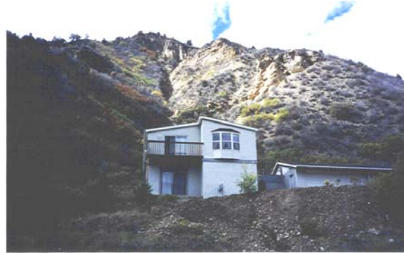
Figure 6: Development has occurred on historic debris fans making many structures vulnerable to flooding by runoff with water and mud.
