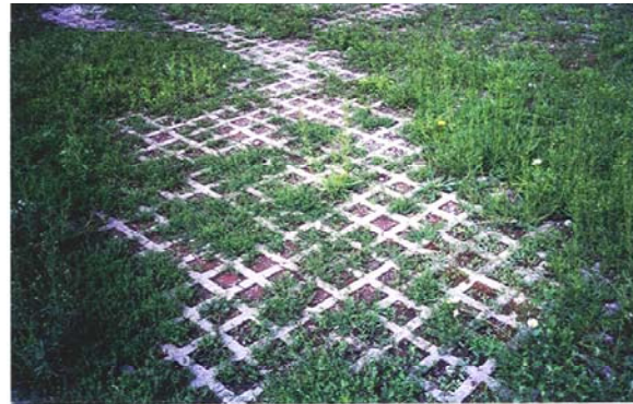
Figure 30: “Porous paving” is encouraged to promote infiltration of stormwater. These blocks can be used in parking lots to reduce the overall site imperviousness and reduce stormwater runoff.
