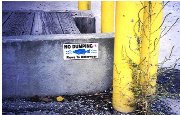
Figure 29: This water quality outlet structure at Safeway informs citizens that anything dumped into the inlet will likely be conveyed directly to the Roaring Fork River. The NPDES stormwater program encourages installation of informational plaques such as this sign.
