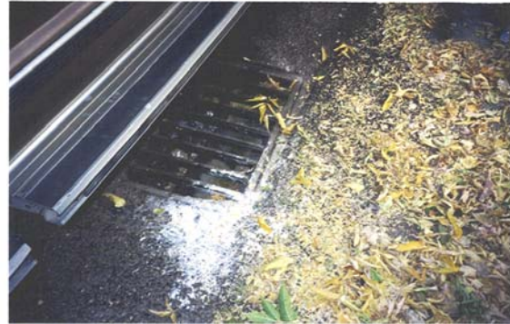
Figure 2: Many citizens do not know that anything discharging into storm drains goes untreated directly into the river. This street inlet was improperly used to dispose of paint.
