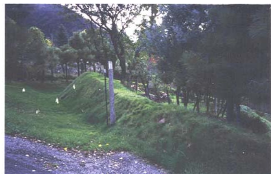
Figure 10: After the severe mud flows in 1977 and 1981, this homeowner constructed a berm to protect his property from damaging runoff.
