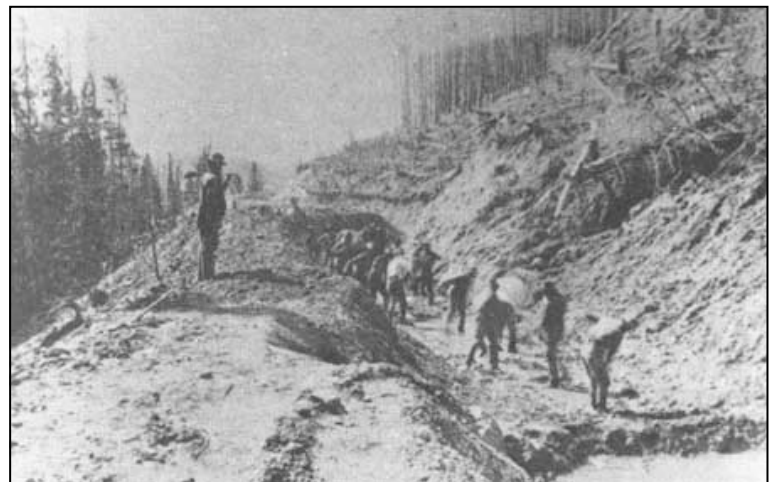
Figure 1. Japanese and Mexican workers dug mile after mile of the Grand Ditch using only picks and shovels (circa 1904). (Fort Collins Museum)
