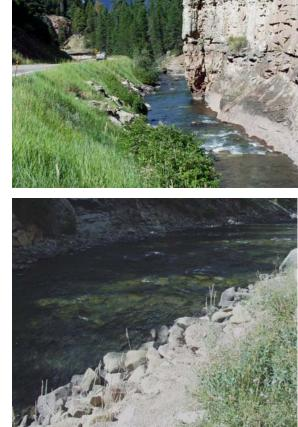
Left: Bedrock controls the right bank but the highway confines the left bank and inhibits meandering. Right: Road-base gravel has been flushed into the stream by runoff, filling pools and embedding cobbles.
