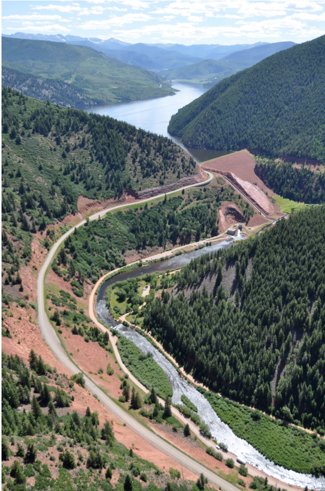
Figure 1. View looking upstream on the Fryingspan River toward Ruedi Reservoir (Photo Credit: USBR)
