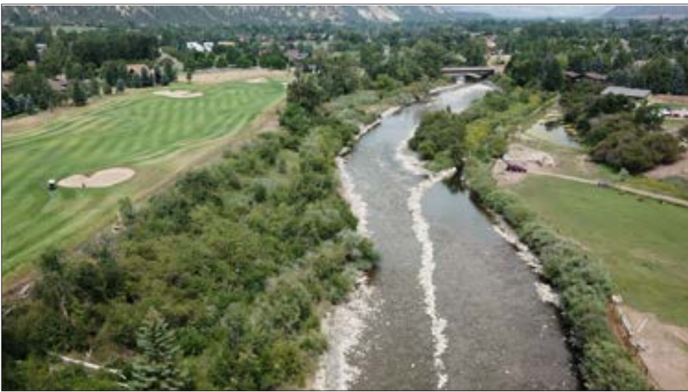
Looking downstream at the Weaver Ditch diversion and project area.
