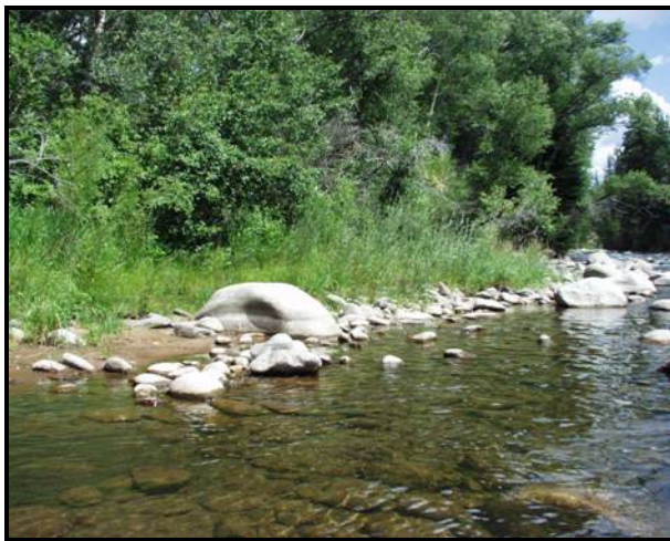
Figure 4.2.9. Reach RF4-7: Removal of native understory shrubs and herbaceous plants have resulted in bank erosion (see upper photo). On the opposite bank, landowners have conserved native vegetation (lower photo), resulting in stable banks and high wildlife value.
