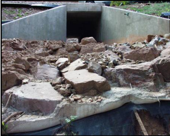
Figure 4.2.11. Wildlife underpasses funnel eroding upland sediment into the river.
