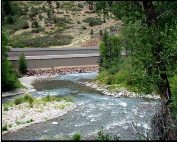
Figure 4.2.8. Highway 82 construction has channelized the river and contributed to instability.
