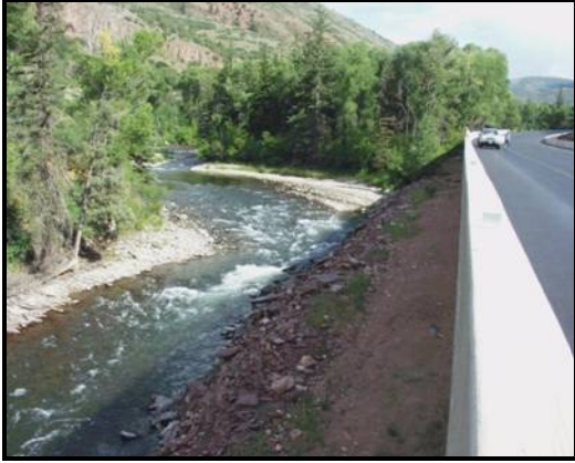
Figure 3.3.13. The development of Highway 82 has caused channelization of the Roaring Fork River.
