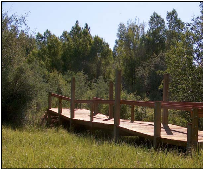
Figure 4.3.9. Boardwalk construction at the USFS Tree Farm to protect wetland habitats (Photo credit: Mark Lacy).
