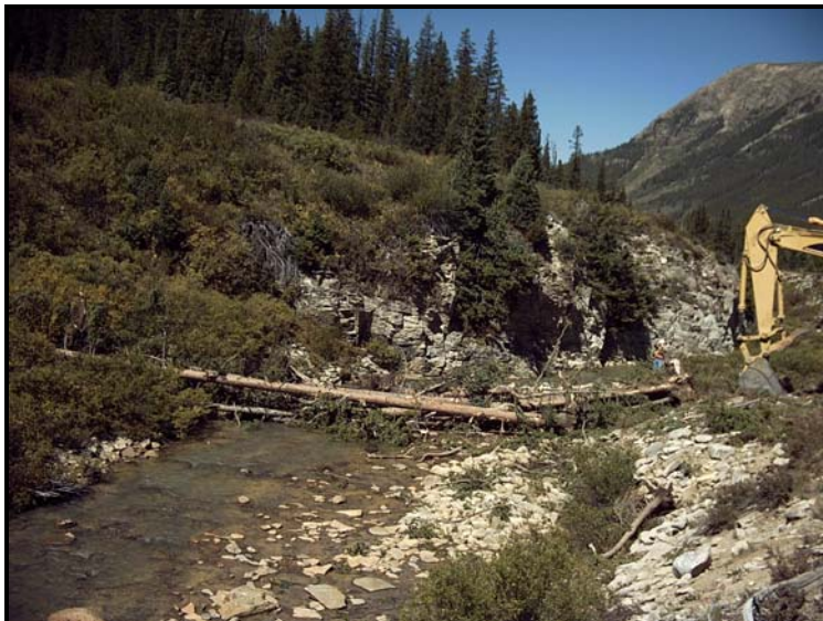
Figure 4.1.24. Large wood replacement project Lincoln Creek, 2004. Upper photo: Before large wood was placed. Lower photo: Wood being placed in stream. Photo credits: Mark Lacy.
