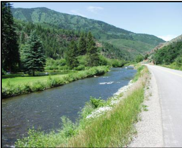
Figure 4.7.17. Fryingpan Road and riprap on the right bank channelizes the stream and inhibits stream processes and functions.
