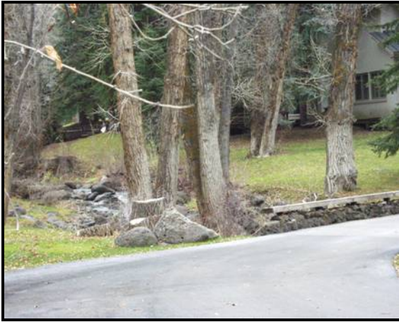
Figure 4.4.14. Residential development and roads in the riparian zone in reach 4M1-5 have altered vegetation and channelized the stream.
