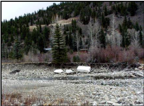
Figure 4.8.23. CR1-2: Channel widening and braiding have occurred from vegetation removal and channel dredging.
