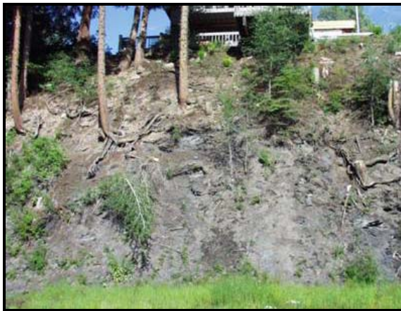
Figure 4.5.9. MA1- 4: Upland development has led to excessive hillslope erosion that moves sediment into the stream.
