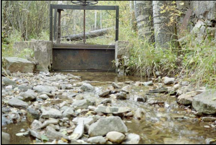
Figure 3.4.13. Stream diversion on West Sopris Creek, September 9, 2006.
