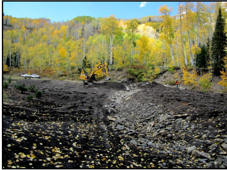
Figure 12. Area 2c alluvial fan during restoration.
