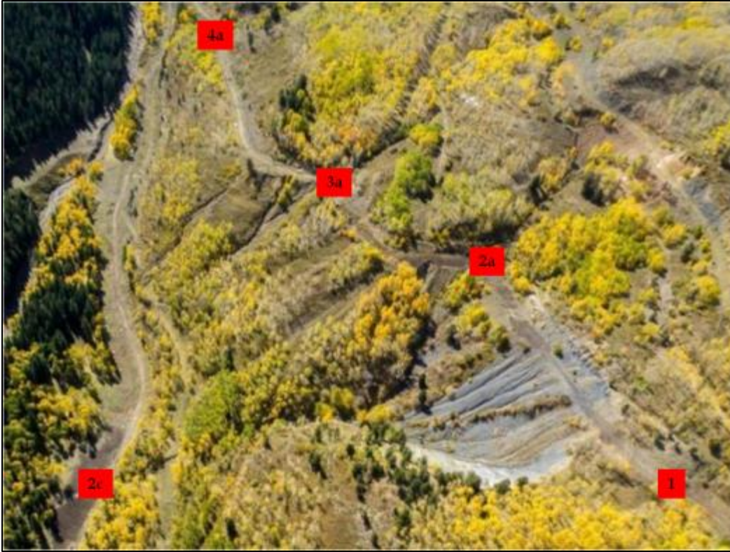
Figure 5. Pilot project area with work ongoing, September 2012 (source: EcoFlight). Note the darkened surface at area 2c (“alluvial fan”), where the largest volume of compost/biochar was applied.
