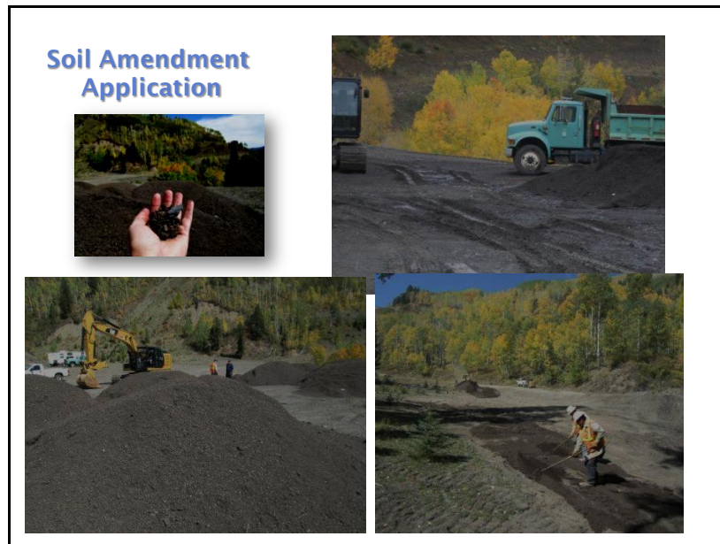
Figure 13. Application of biochar/compost and compost only soil amendments in treatment areas. Top left photo is a close up of biochar. Piles in photos are compost/biochar blend.
