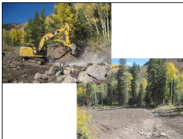
Figure 11. Area 2c alluvial fan during restoration.
