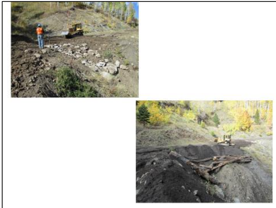
Figure 7. Area 2a during restoration.
