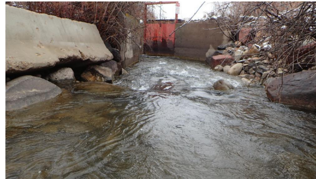
**December 2020:** The current Weaver Diversion headgate, consisting of concrete barriers and outdated gate infrastructure. Portions of the Weaver Diversion will be rebuilt with native materials and will be enhanced by two new, modern headgates, funded by the Pitkin County Healthy Rivers Board. The new headgates will increase the ability to control water entering the Weaver Ditch and will have the ability to be retrofitted with an automated system in the future.
